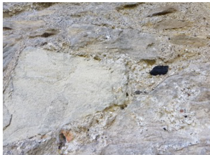
The remains of lime mortar and harl at Kinneil House, with evidence that coal was used to burn the limestone. Photo Nicola Ashurst
