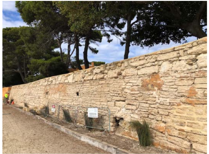
Removal of acrylic paint and cement render, the raking out of the joints to take new lime pointing. Note: the wall was extended approximately 800 mm in the 1960s Picture Colgan Industries Pty Ltd
