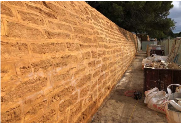
John Kelly, one of Colgan Industries Head Stone Masons replacing deteriorated stone with new facing. Photo Colgan Industries Pty Ltd
