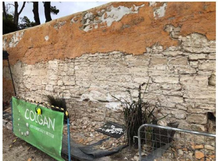
Cement render being removed Photo Colgan Industries Pty Ltd
