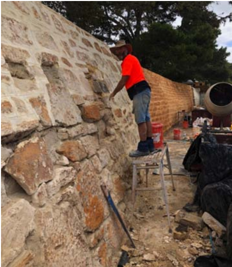
John Kelly, one of Colgan Industries Head Stone Masons replacing deteriorated stone with new facing. Photo Colgan Industries Pty Ltd
