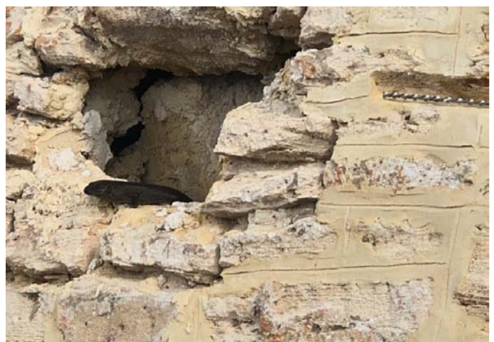
Friendly skink, freshly applied hot mixed lime and a Helical Bar Tie on delaminating on skin of outer facing wall. Photo Colgan Industries Pty Ltd
