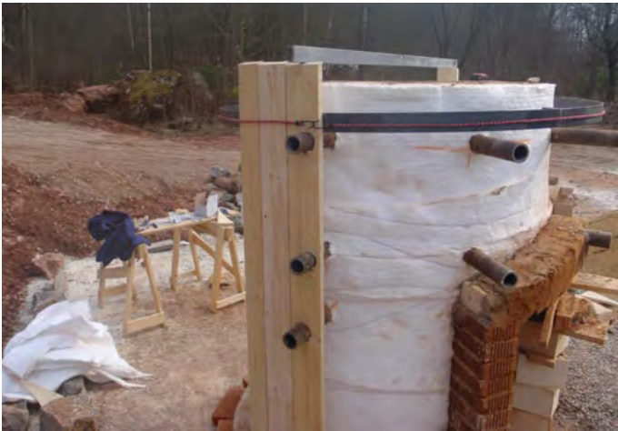
Prague kiln under construction Photos Jan Valek
